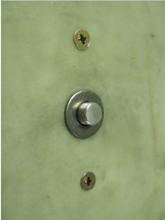
Set at 3/16" above the surface the button is flush when the latch releases.
